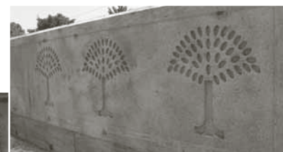
Look what's on the new walls of the Southfield Freeway!
