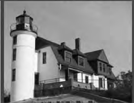
PT. BETSIE LIGHTHOUSE, Frankfort, MI 2010 Governor's Award for Historic Preservation
