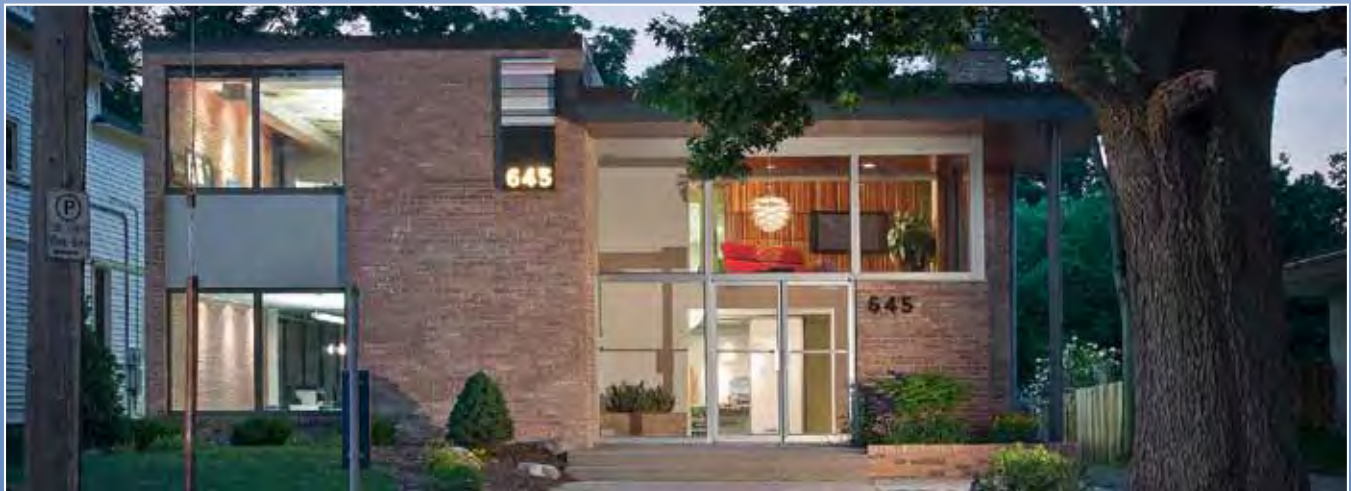
645 Cherry (aka New York Life Insurance Building) Grand Rapids, MI Submitted by: Lott3 Metz / Chuck Heiney photographer
